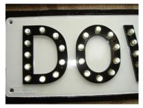
Picture 1 **reflective studs** - shows how the new reflective studs (all studs on all plates are new) work. These studs came from The Reflective Road Stud Company which was founded by the inventor of the 'cats eye' Percy Shaw. They arrived wrapped in newspaper dated from the early 1950's so it's safe to say they are original parts for your signs.
